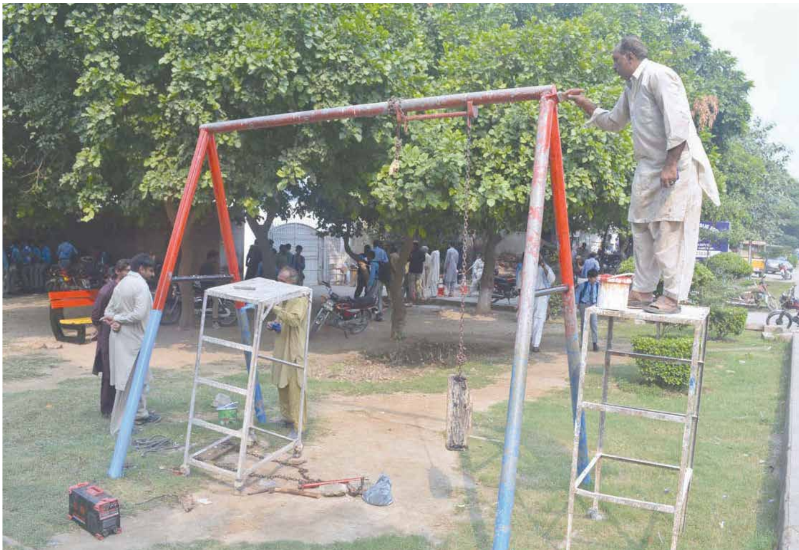
SARGODHA: Workers busy in maintenance work of a swing installed near Divisional Public School at Club Road.
