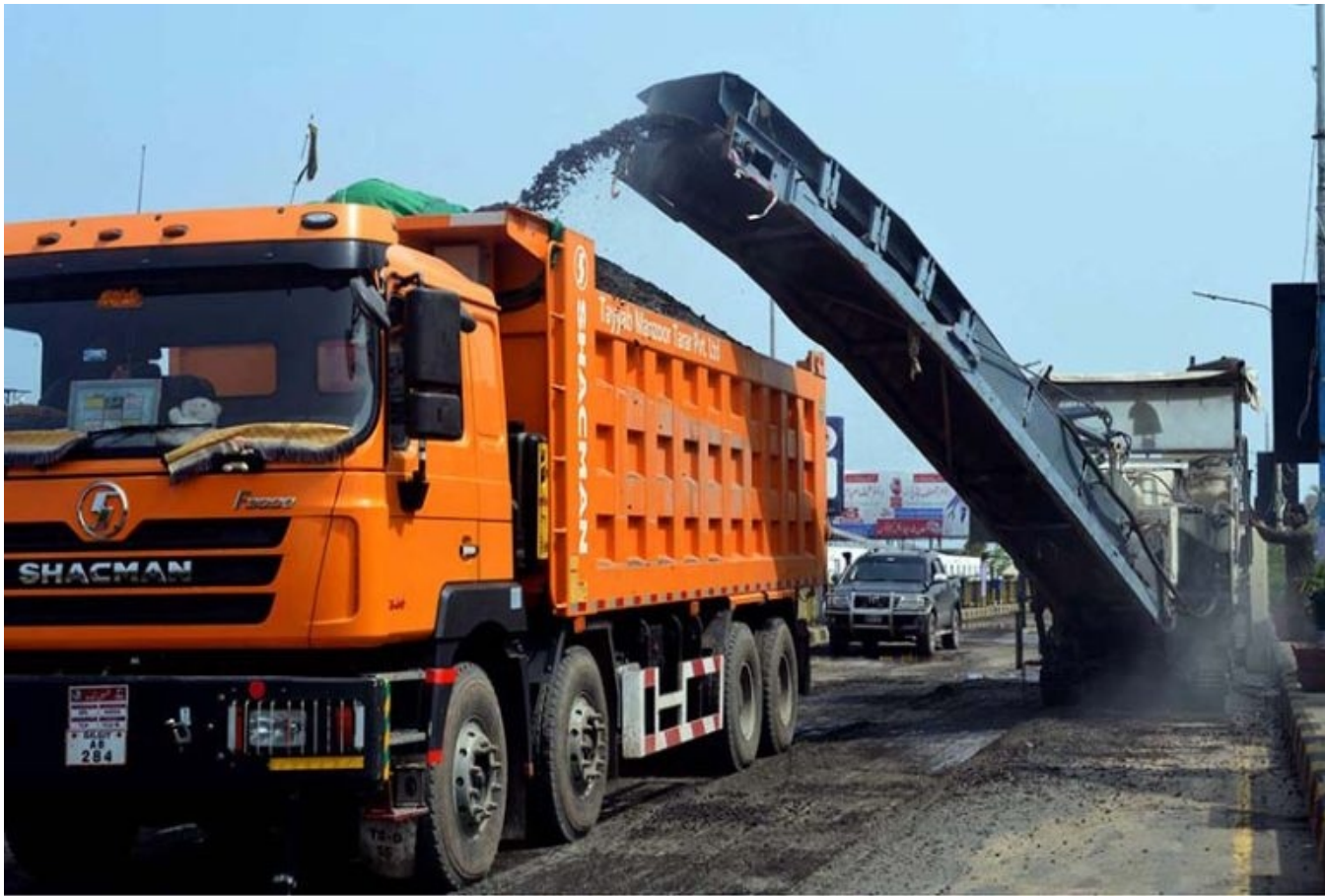
A milling machine loads asphalt material onto a truck during road construction work
